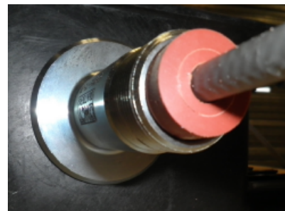
Push 1 piece of Seal into place
